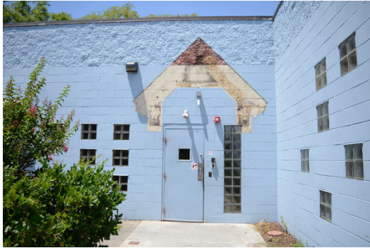
Family Shelter Exterior
